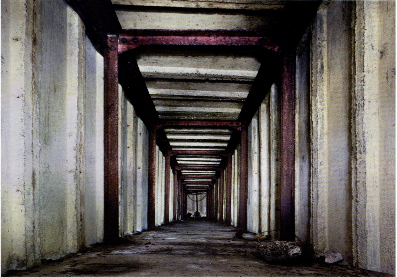
One of the passages in the recently re-discovered air-raid shelter in Carshalton Park, Carshalton, Surrey. Photo Nick Combes
